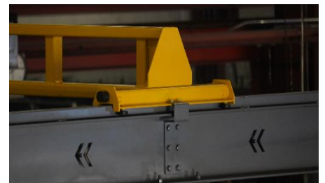
Image 5B. Bridge Lock Plate
