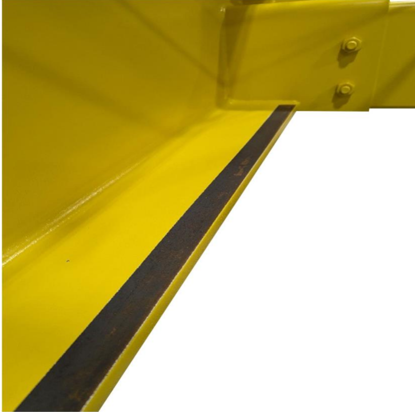
4.4.1 Taped Off Section on Crane
